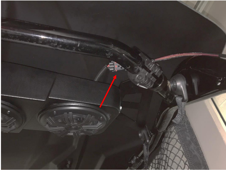
Figure 10: Chassis harness connected and routed over front roll bar.
