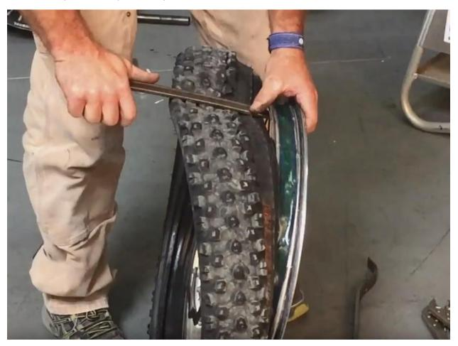
The wider of a section you can get started off of the rim, the easier the tire will come off when you apply pressure.
